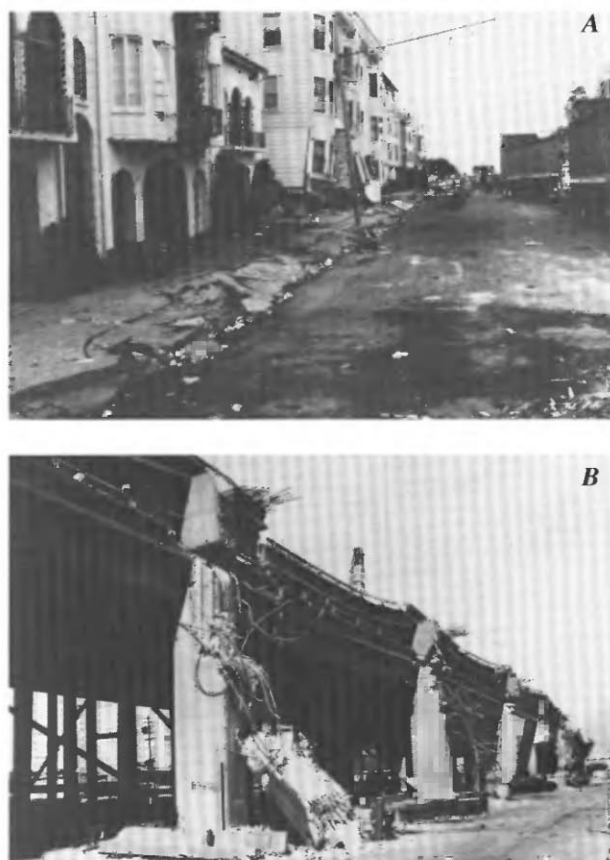
FIGURE 6.10.—Damage in October 18, 1989, Loma Prieta earthquake occurred at distances as far as 100 km from the epicenter in areas underlain by water-saturated, unconsolidated material. A , Liquefaction-induced ground failure in the Marina district of San Francisco (top) was restricted to land reclaimed from the San Francisco Bay. B , In Oakland, the second deck of Interstate Highway 880 collapsed onto the first deck. Here, poor design was the principal culprit, although failed section sits atop estuarine sedimentary deposits that amplified the shaking.
