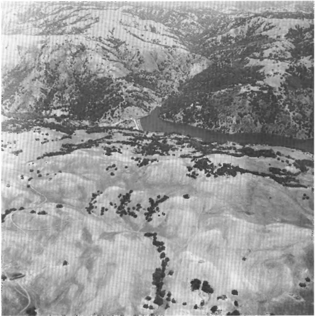
FIGURE 2.35.—The Coyote Lake Reservoir lies in a topographic trough along the Calaveras fault a few kilometers east of Morgan Hill, Calif. View eastward across fault.
