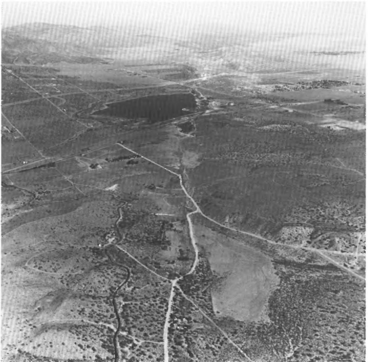
FIGURE 2.29.—The Palmdale Reservoir lies along the San Andreas fault north of the San Gabriel Mountains. The Mojave Desert is to northeast (right), and a series of ridges lies between the fault and the desert basin. View northwestward.
