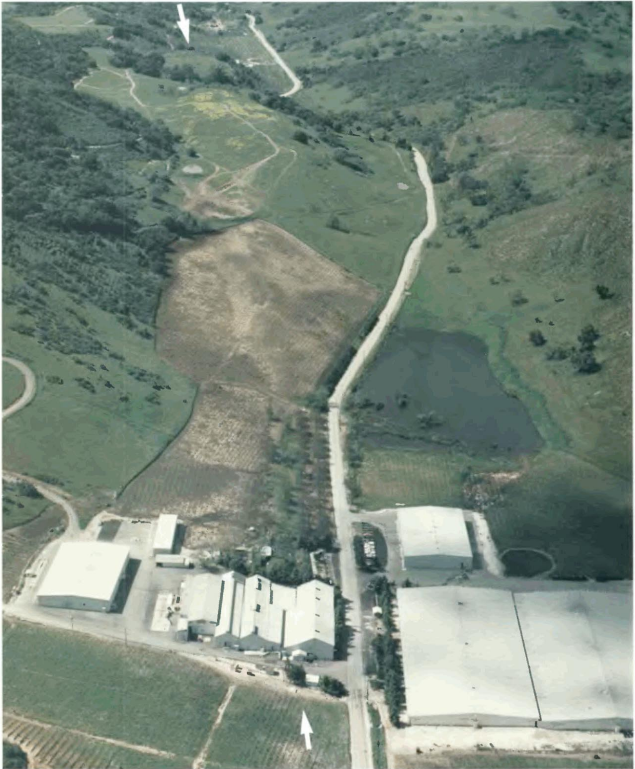
FIGURE 2.14.—Fault creep on the San Andreas fault was first reported at the Paicines Winery south of San Juan Bautista in 1960 by Steinbrugge and Zacher (1960). Fault trace (between arrows) passes under winery building, and walls of building are continually being displaced. View northwestward.
