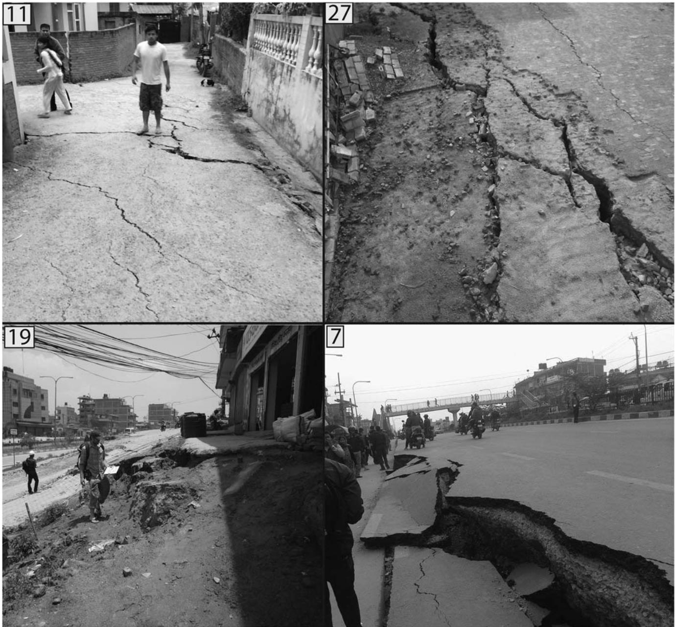
▲ **Figure 5.** Example photographs of the newly developed fracture set in Kausaltar. The number in the upper left corner gives the location number indexed to the map of shown in Figure 4a. Additional color photographs of Kausaltar fractures are provided in the (©) electronic supplement.
