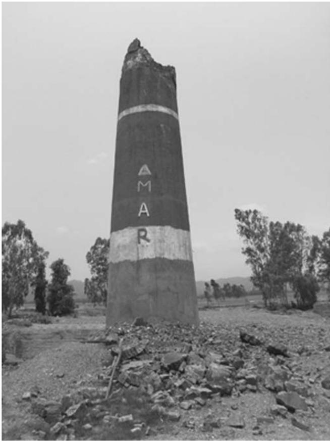
▲ **Figure 6.** Representative photo of a failed chimneystack located on the Indo-Gangetic Plain.
