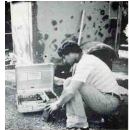
Austin Wilson installing portable seismograph with the Lab trailer in background. Circa 1980. Photo from Mackay Miner 1983.
