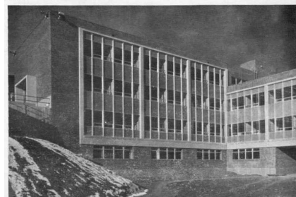
Mines wing of new James G. Scrugham Engineering-Mines Building.
