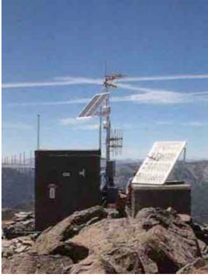
Installation and modifications of communications stations is challenging prospect on remote mountaintops of Nevada.
